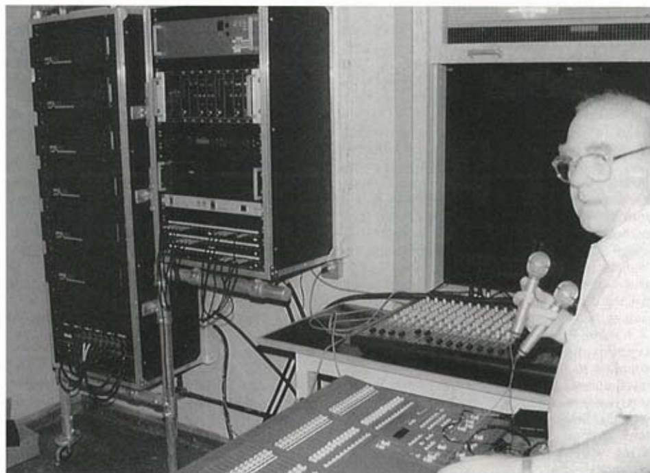
A Strand MX provides control for lighting, whilst to its right, an Allen & Heath SC+ mixes the sound. In the background are the Citronic amps and ARG digital delay unit.
